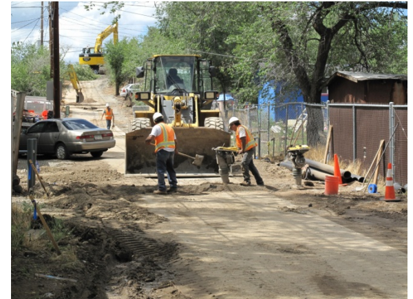
Small Water Mains Phase 1
