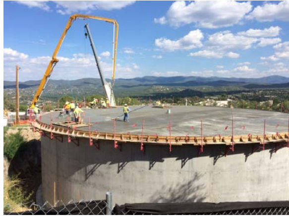
Zone 27 Tank Construction
