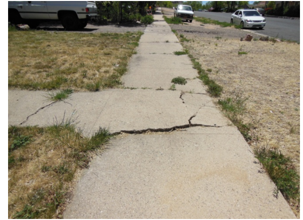
Sidewalk Repair Project
