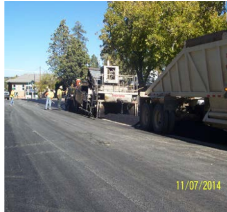
Park Avenue Paving
