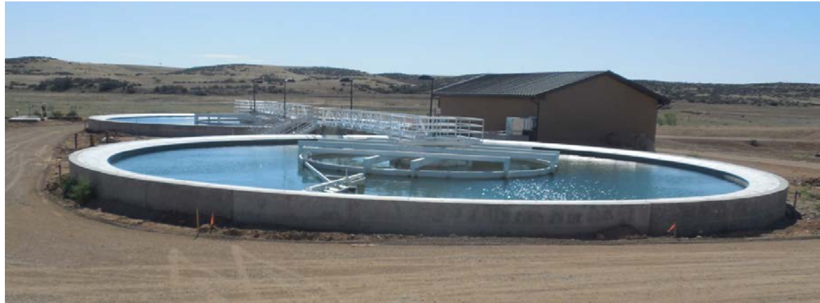
Airport Wastewater Reclamation Facility Phase 1
