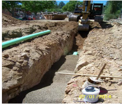
Park Avenue Sewer Line
