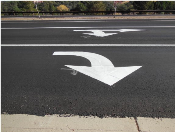
Lee Blvd After Resurfacing
