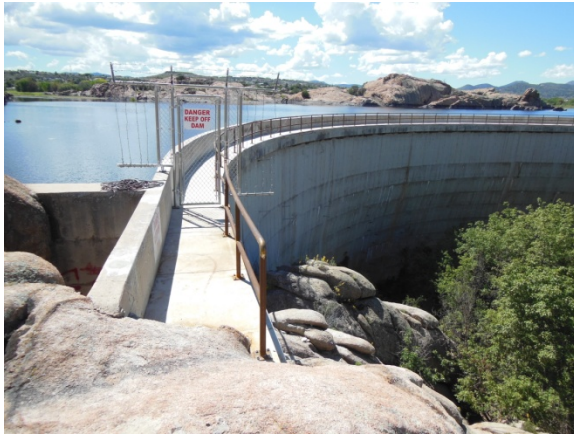
Willow Creek Dam Repairs
