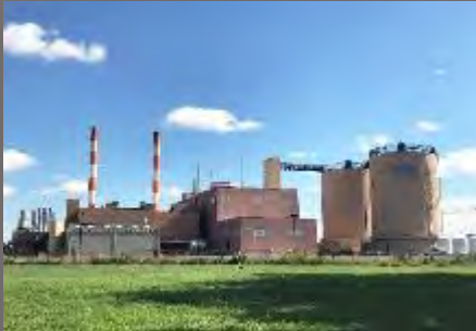
Green Bay, WI 2 – 2.0 MG Digesters New Water WTP
