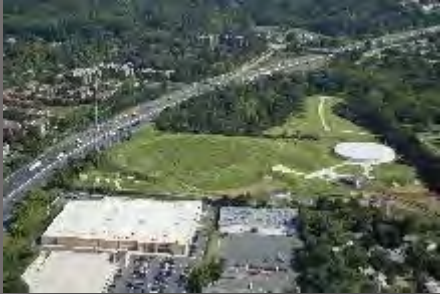
Pikesville, MD 1 – 15.3 and 1- 5.07 MG Ground Storage Tanks Baltimore County Dept. of Public Works
