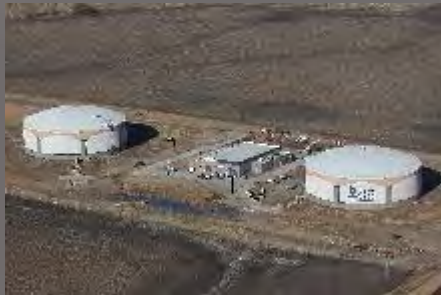
TEA, SD 2 – 7.5 MG Ground Storage Tanks Lewis & Clark Regional Water System
