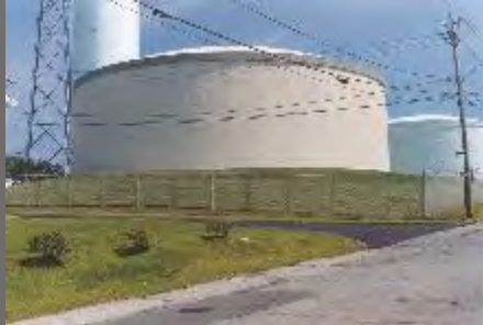
Woonsocket, RI 3.0 MG Water Storage Tank City of Woonsocket
