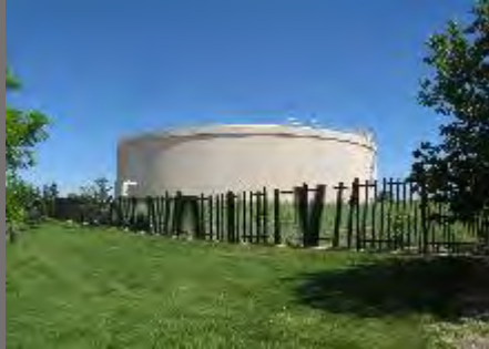
Westminster, CO 3.8 MG Ground Storage Tank City of Westminster
