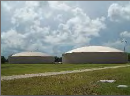
Spears Road, TX 2 – 10.25 MG Water Storage Tanks North Harris County Regional Water Authority
