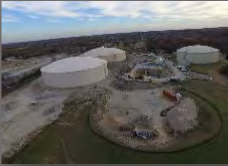
McKinney (University), TX 10.0 MG Water Storage Tanks City of McKinney
