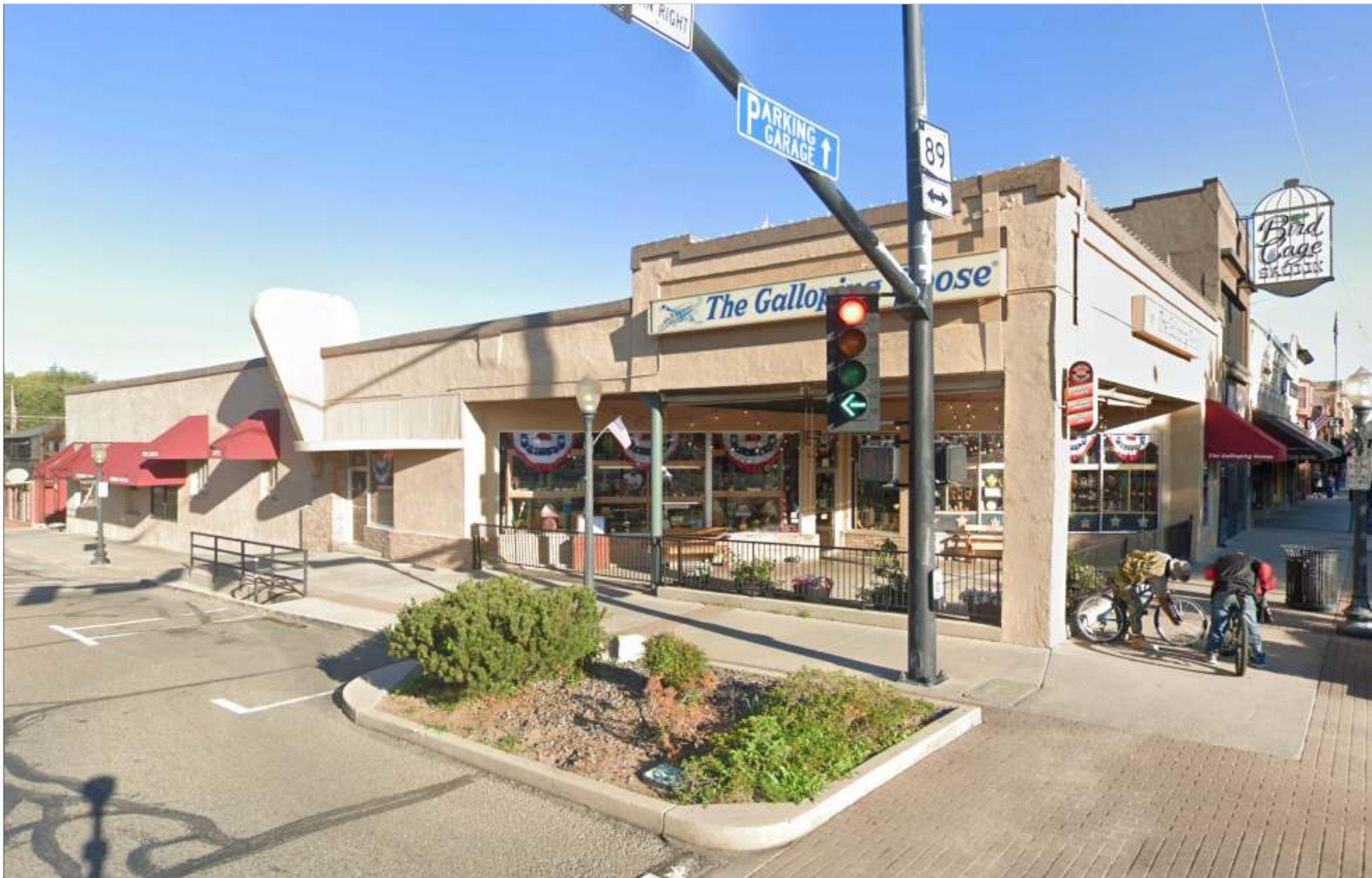
1 EXISTING VIEW FROM SE CORNER LOOKING NORTHWEST SCALE: N.T.S.
