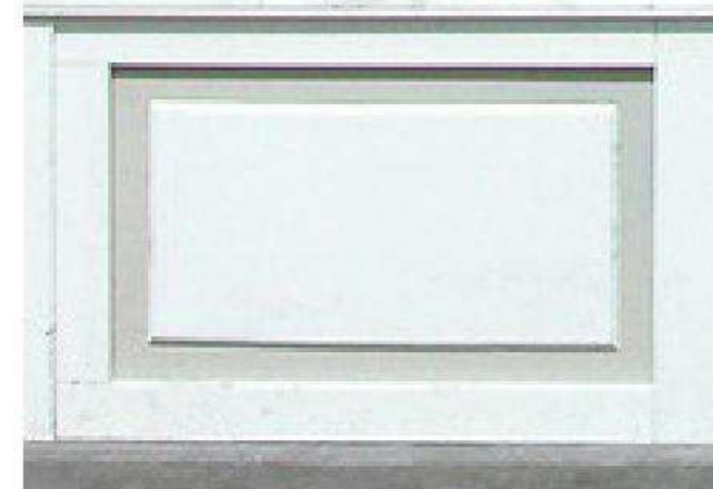
STOREFRONT BULKHEAD PANELING - SW 7005 PURE WHITE
