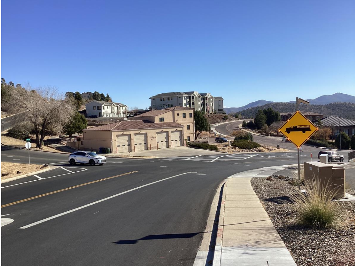
Lee Blvd Fire Station and Intersection Striping
