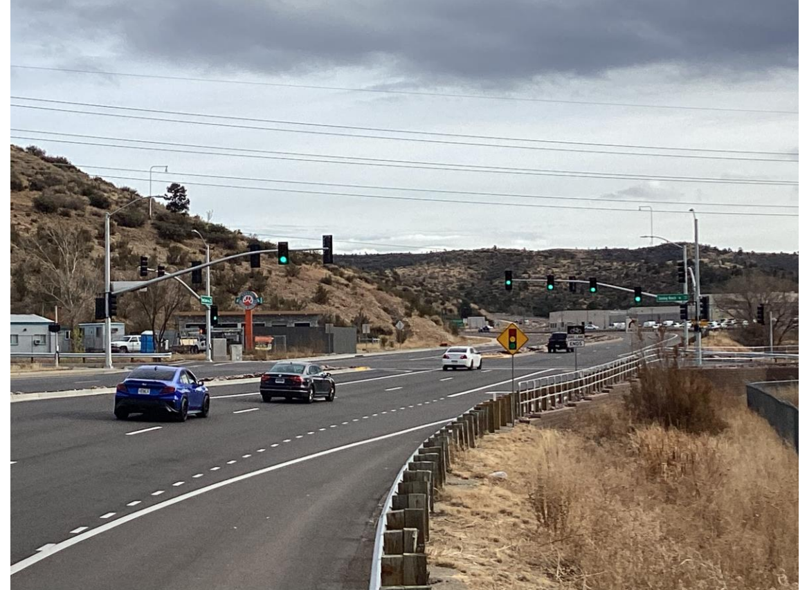
Prescott Lakes Parkway at Sundog Ranch Road Traffic Signal/Intersection Improvements
