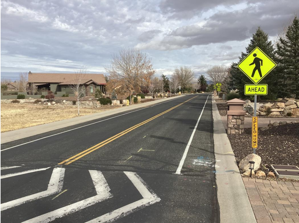
Robin Drive/Clearwater Drive Traffic Calming
