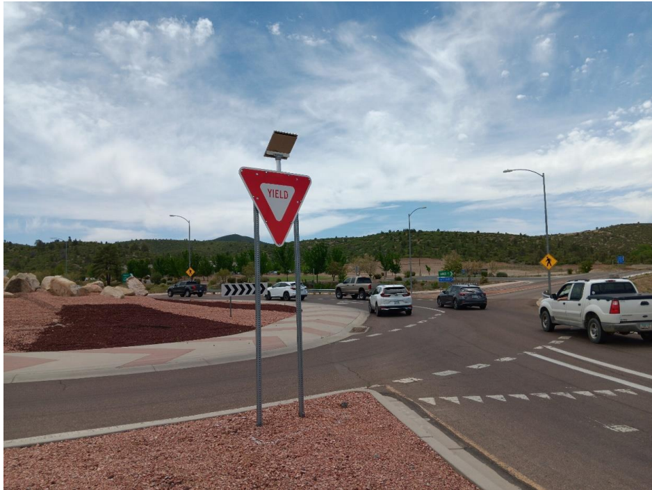
Roundabout LED Flashing Yield Signs
