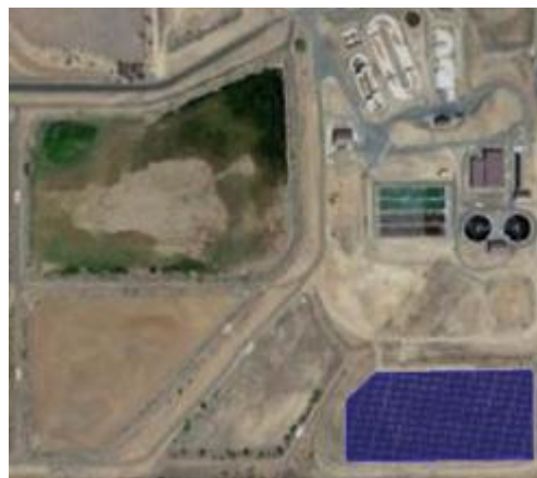
Figure 11. Possible Ground-Mount Solar Location at Airport WWTP
