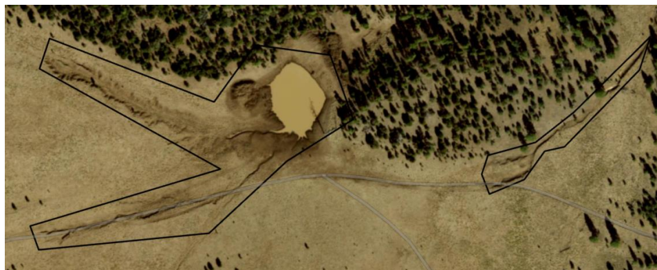
Figure 30 Head cutting and erosion around the stock tank and roads on JJJ Ranch.
