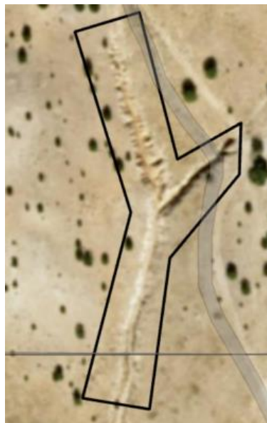
Figure 35 Headcut emanating from road drainage on Chino Grande Ranch LLC's property.
