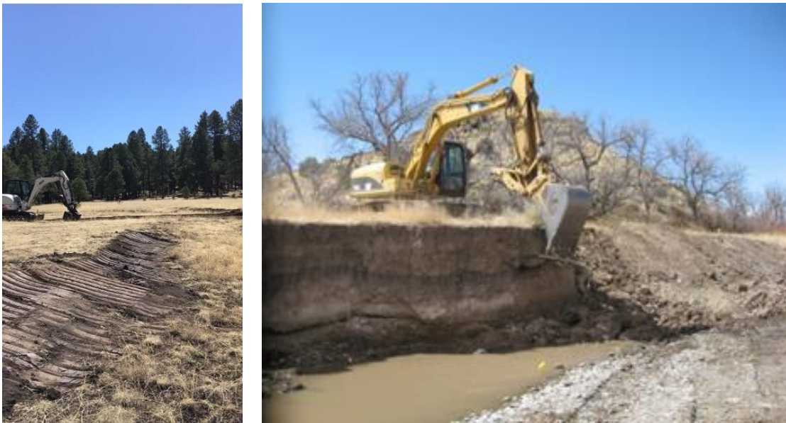
Figure 43. Bank sloping practices in various areas within Northern Arizona. Note the use of excavators for these photos; however, bank sloping practices can be scalable and completed by hand crews.
