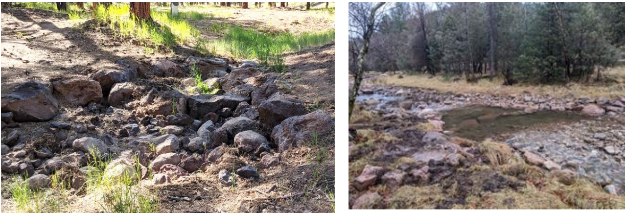
Figure 47 Cross vane weir in an ephemeral channel (left) and in a perennial channel (right).
