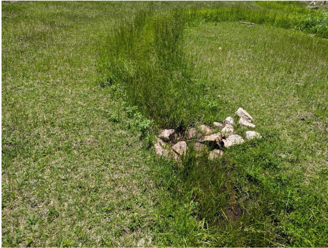
Figure 45 One-rock dam constructed in an incised meadow channel, aggrading and retaining water upstream. In the photo, water flows from top to bottom.
