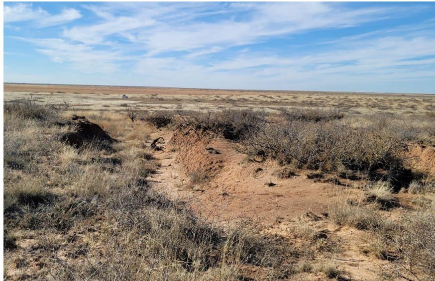
Figure 49 Example of an incised gully through grassland, prior to plug and spread construction.
