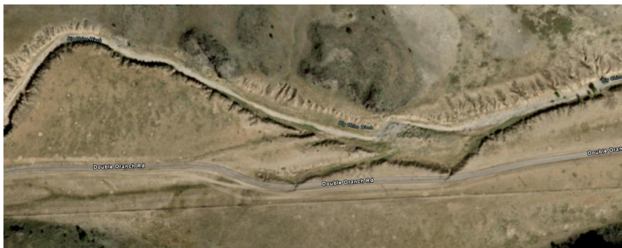
Figure 39 Bank erosion and head cutting along Big Chino Wash on Chino Grande LLC's property
