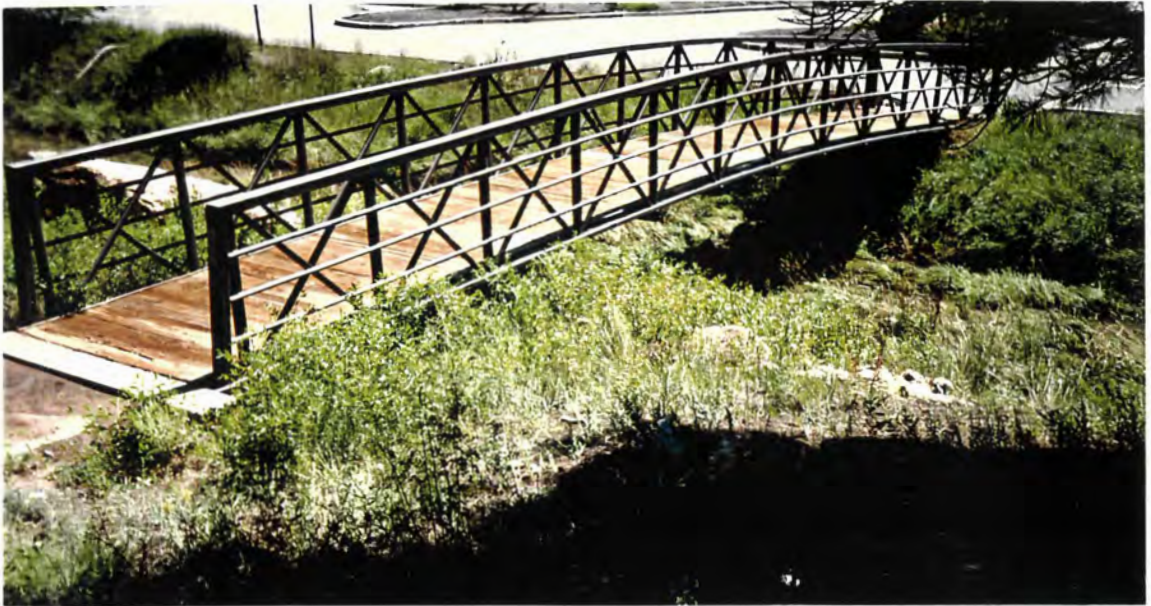
Sample Trail Bridge
