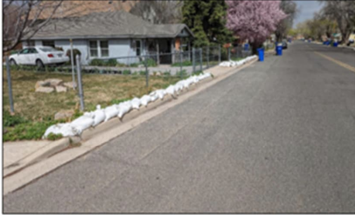
Photograph 1-4. Flood mitigation measures (sand bags) by resident. Located on Lincoln Avenue, south of Merritt Street.
