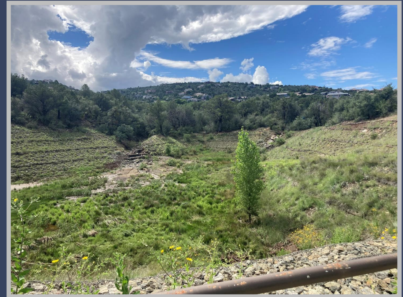
Acker Detention Basin
