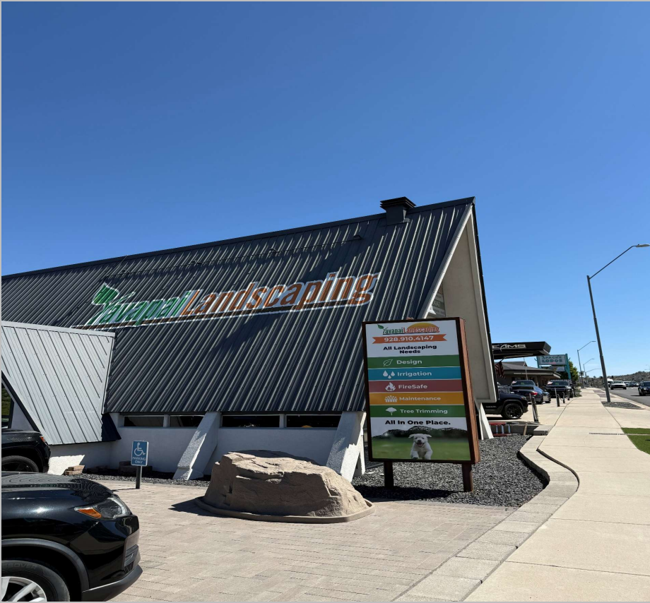
VIEW OF PROJECT AREA - FACING EAST
