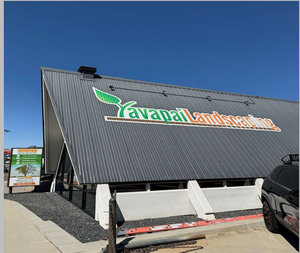
VIEW OF PROJECT AREA - FACING WEST
