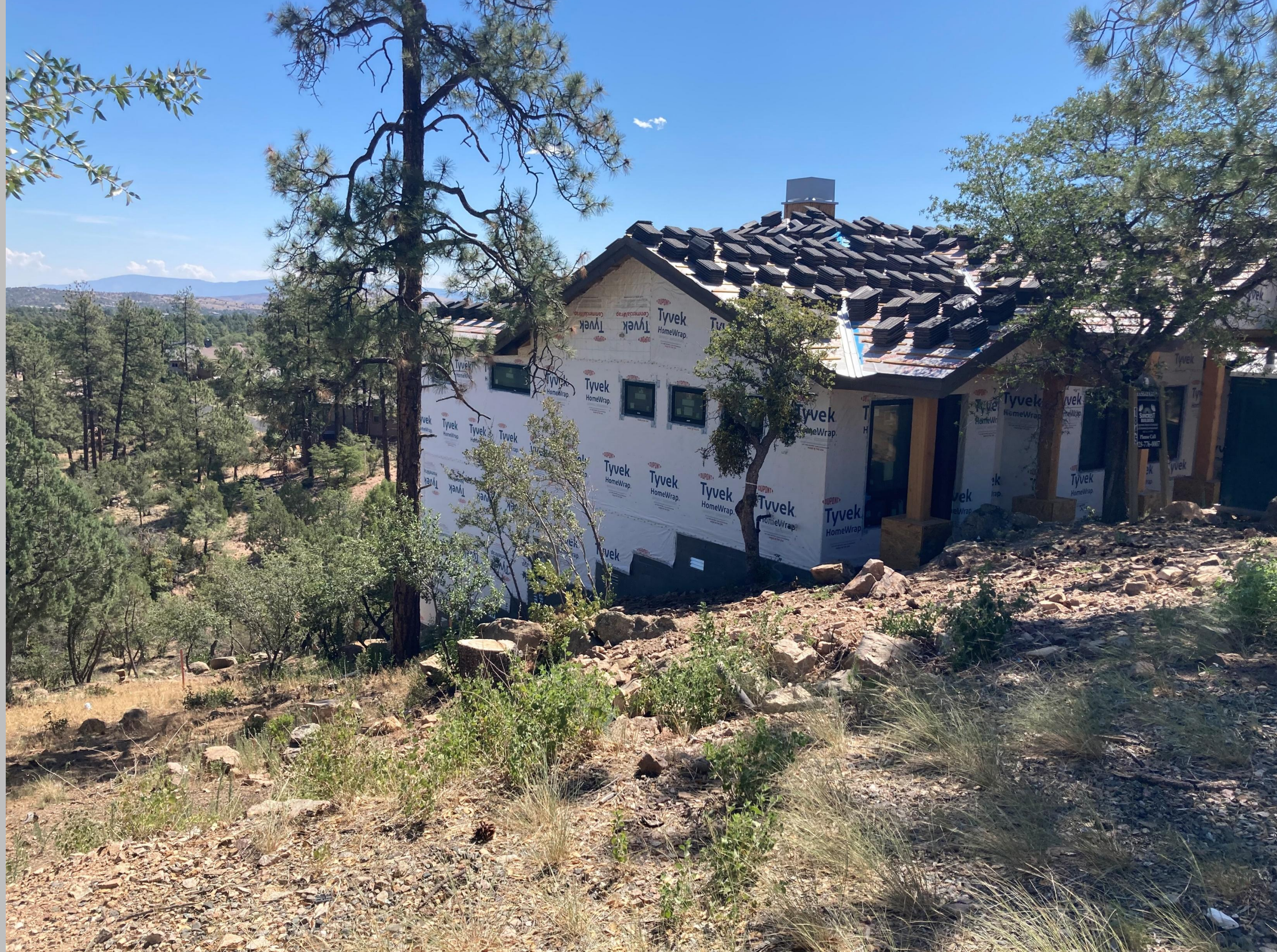
House being constructed next Door to subject parcel
