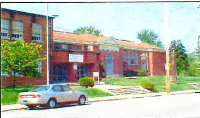
The school prior to rehabilitation.
