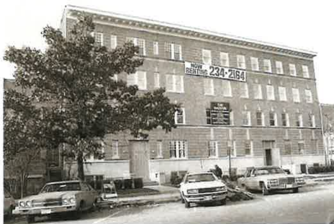
This early twentieth century apartment building was actually constructed as two buildings of harmonious but slightly different design.
