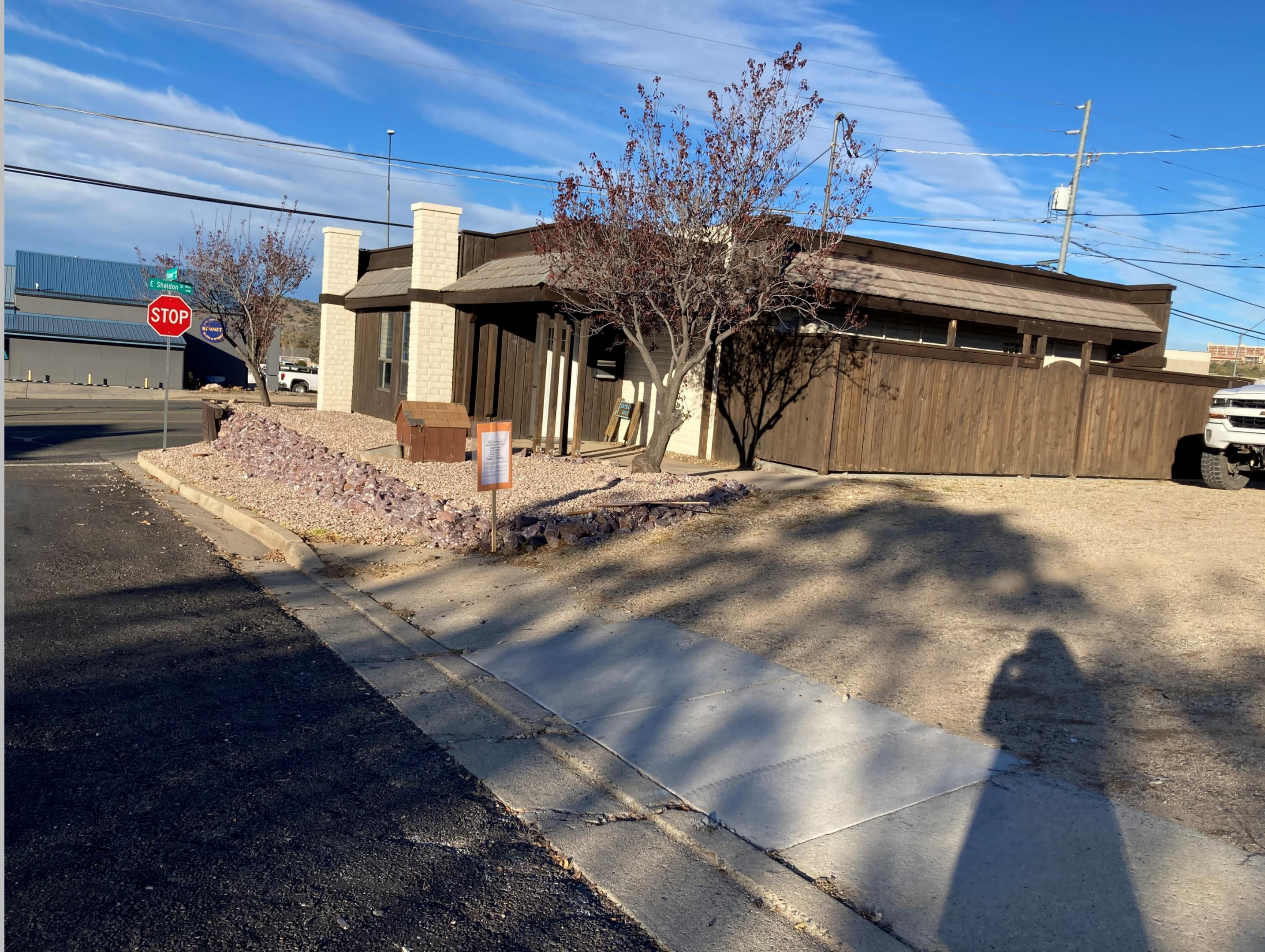
Rear and side of building
