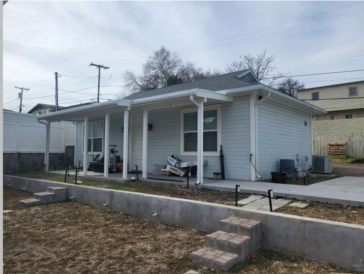
EXISTING GUEST HOUSE – REAR OF PROPERTY
