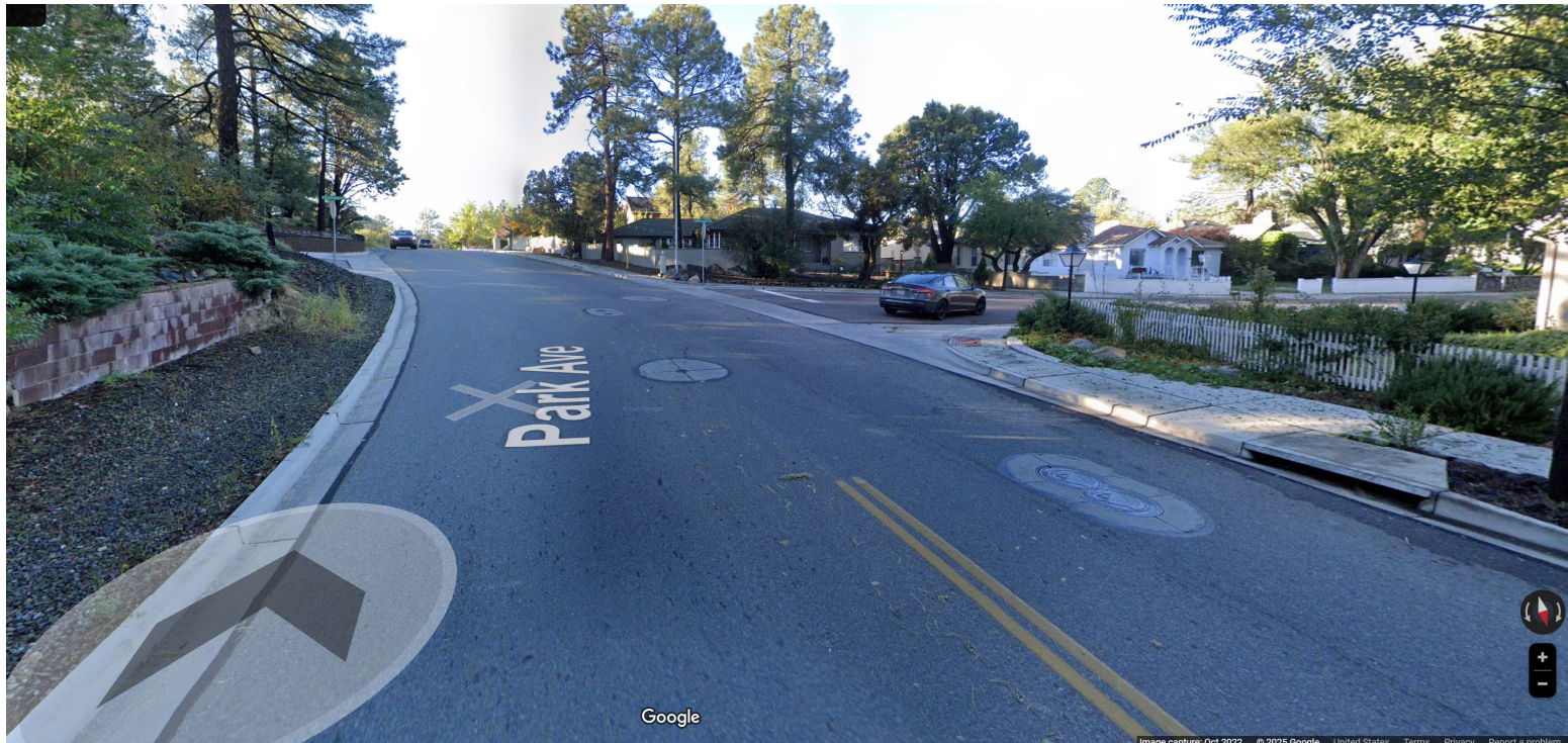
Example of Limited Sight Visibility at SB Park Ave. near Country Club Drive
