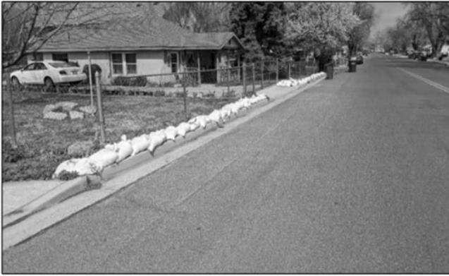
Photograph 1-4. Flood mitigation measures (sand bags) by resident. Located on Lincoln Avenue, south of Merritt Street.
