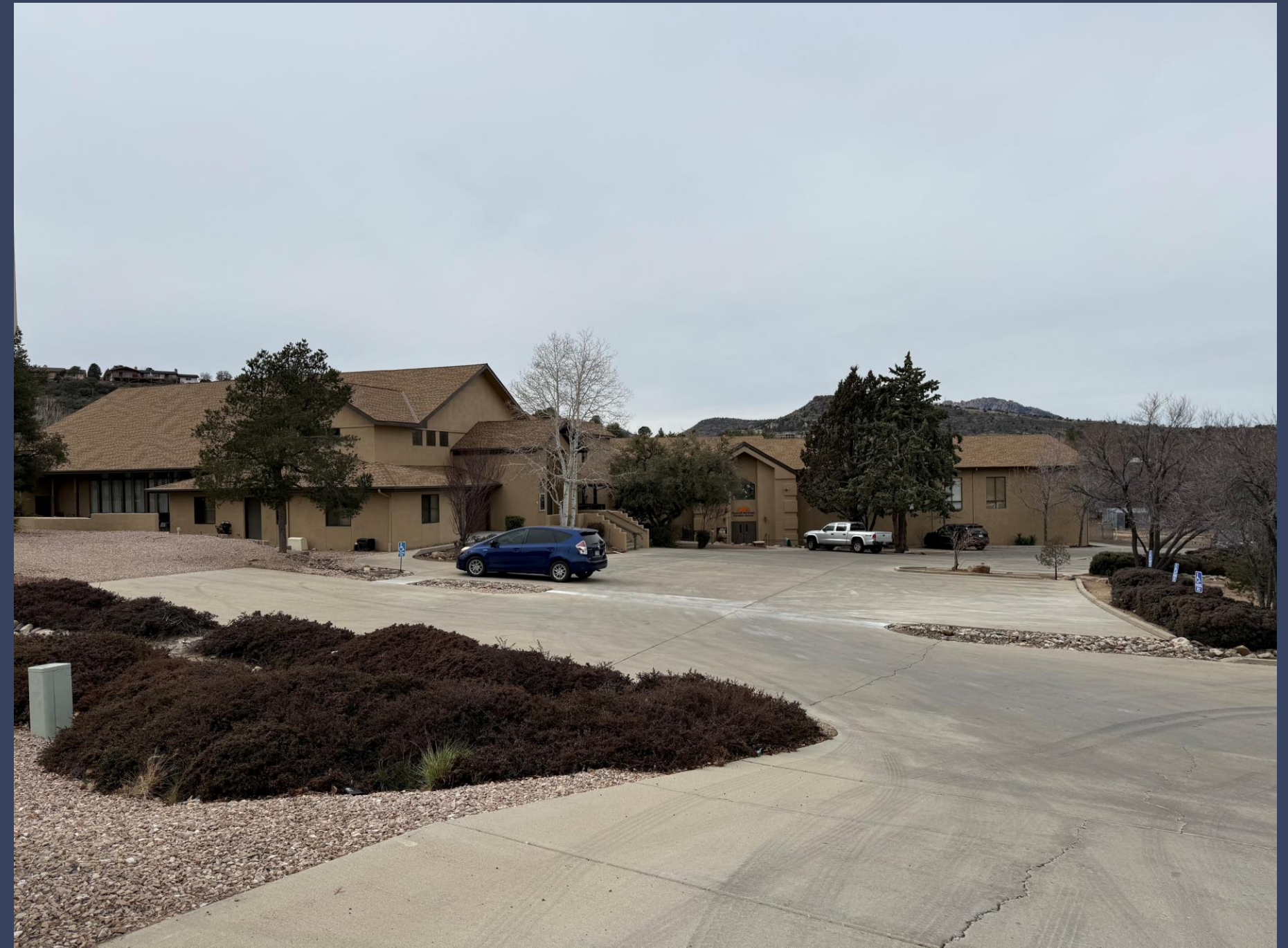
(EXISTING BUILDINGS AND PARKING – FACING WEST FROM WILLOW CREEK ROAD)
