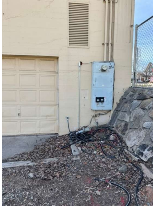
Figure 5 – Location of HVAC Mini Split at the Locker Rooms
