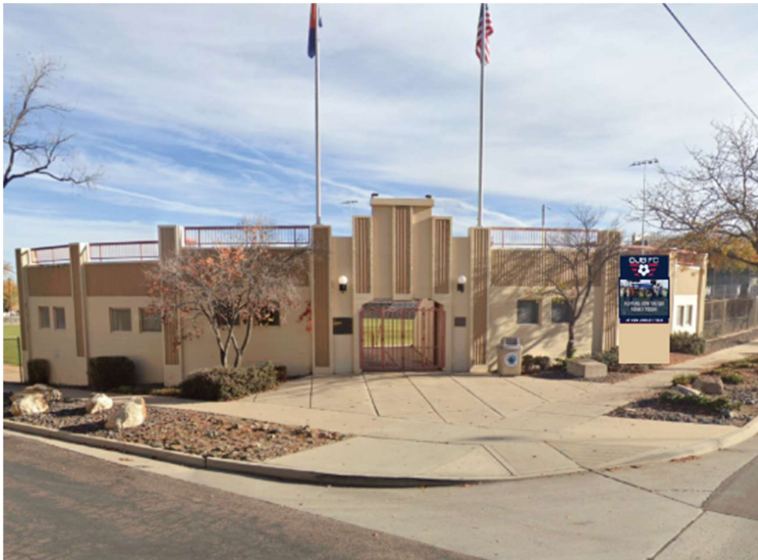
Figure 2 – New Digital Sign at Gurley & Washington Street
