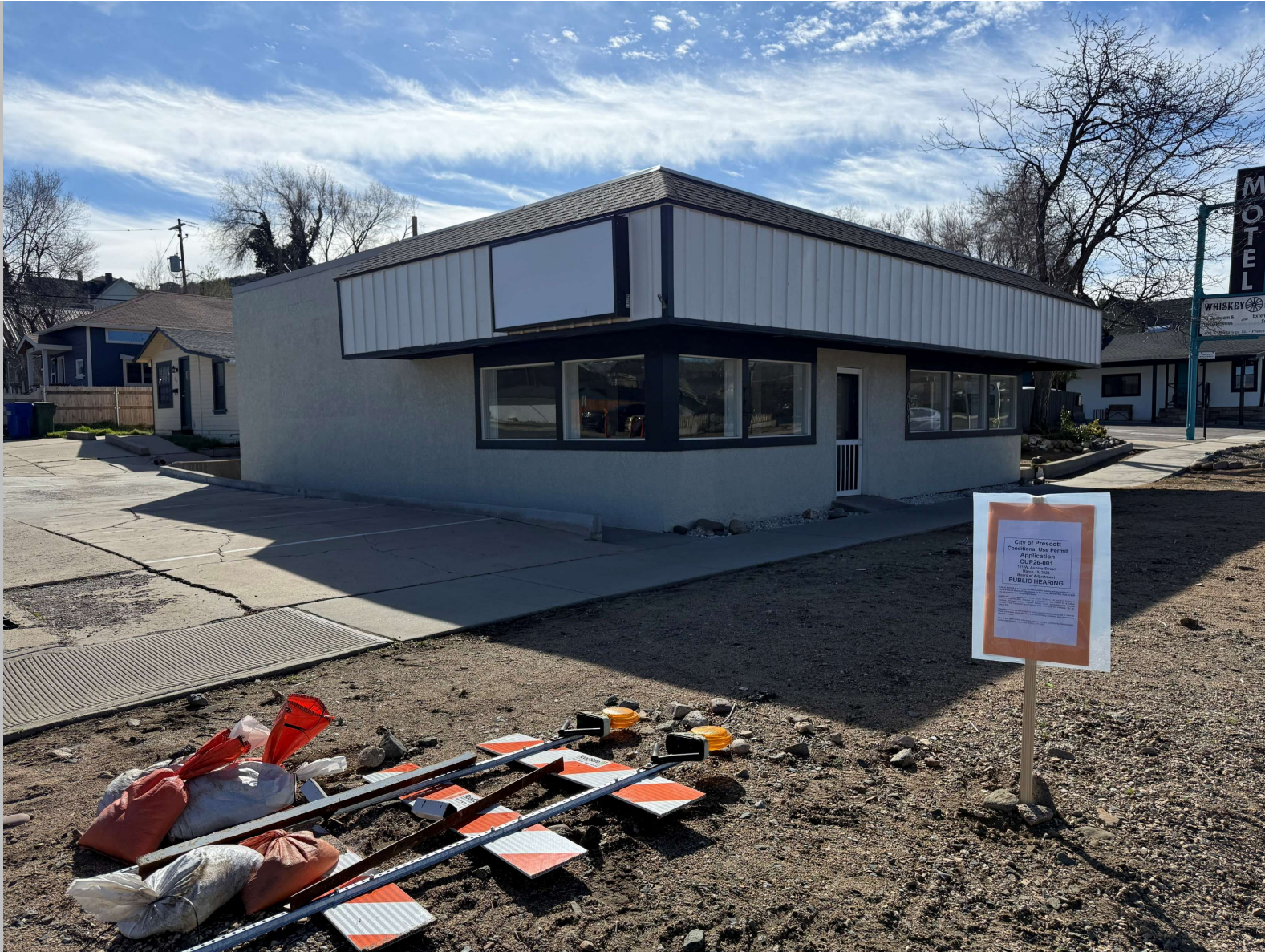
Front & Side of Building (Corner of Montezuma St. & W. Aubrey)
