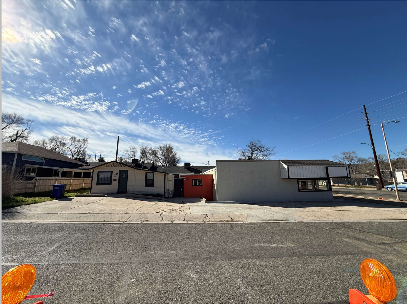
Side of building with parking area (West Aubrey Street)
