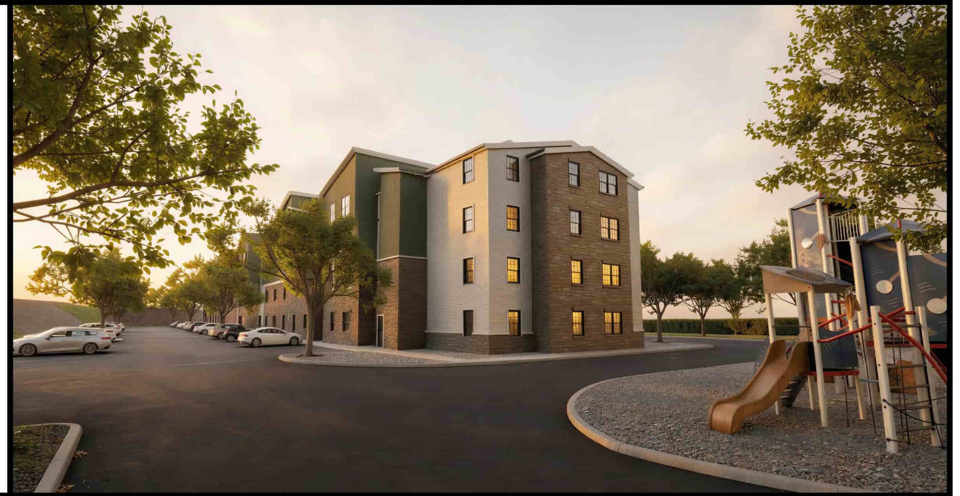
PHOTO BELOW: NORTH ELEVATION FROM PARKING LOT
