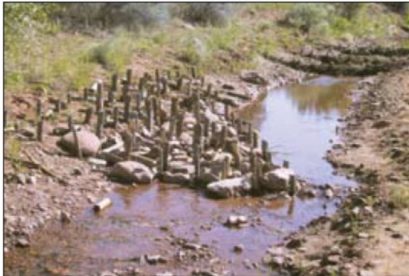
Picket Baffle filled with rocks, Galisteo Creek, NM. (Photo courtesy of Earth Works Institute.)
