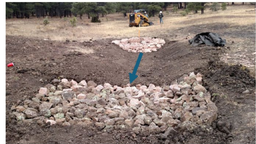
Figure 6. Example of a Zuni Bowl and one-rock dam built in series to arrest a headcut and begin channel aggradation. Arrow indicates direction of flow.
