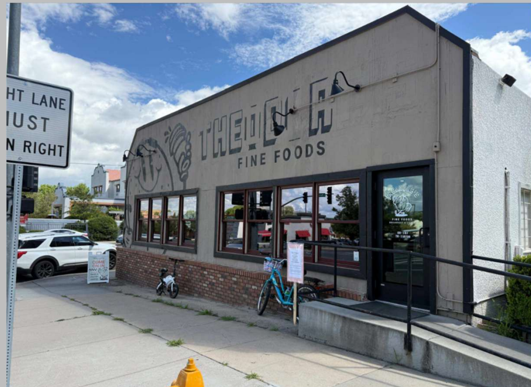
FRONT OF PROPERTY – FACING NORTH FROM N MARINA ST.
